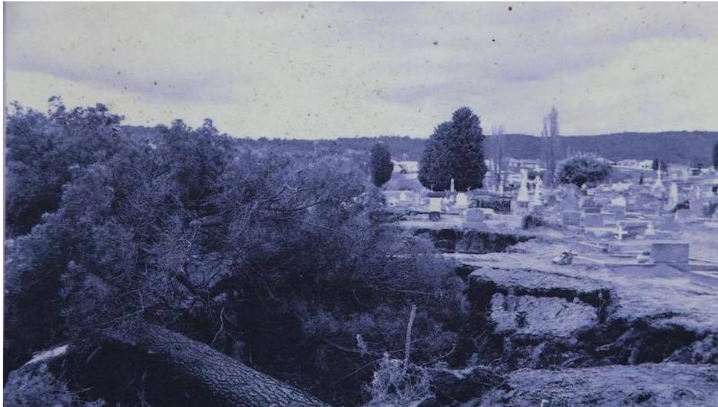
Figure 20: Damage to Riverside Cemetery after 1974 flood (Source: ABC News, 2017)
