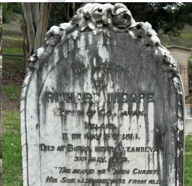
Figure 77: An example of marble discolouration and soiling
