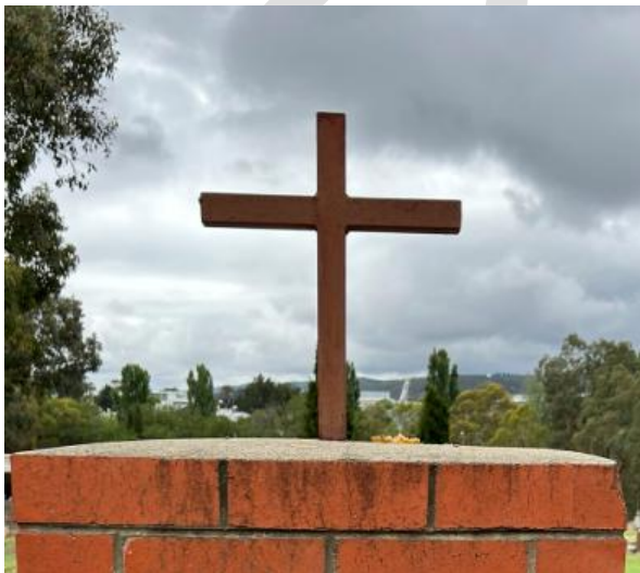
Figure 39: Close up image of the cross embedded in the top of the piers
