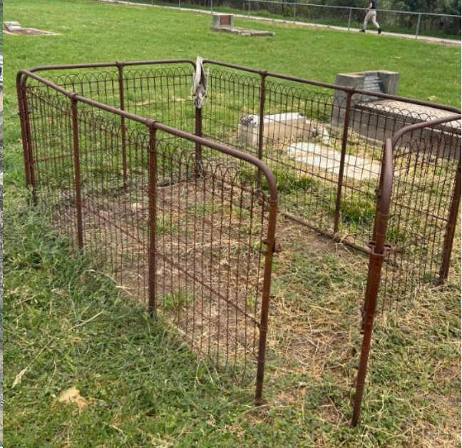
Figure 99: Example of fencing installed directly into the ground
