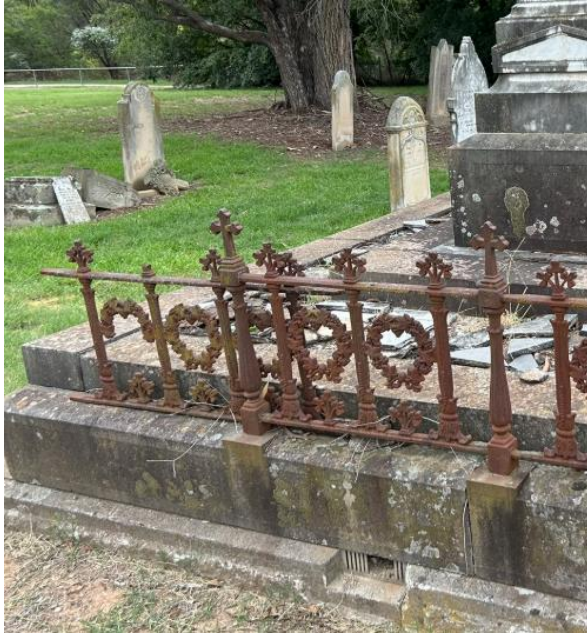
Figure 84: Example of ornate ironwork, some of which has been displaced
