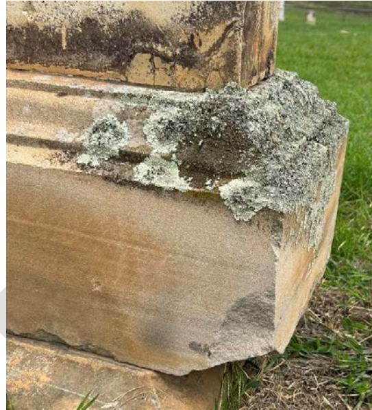
Figure 67: Biological growth on sandstone
