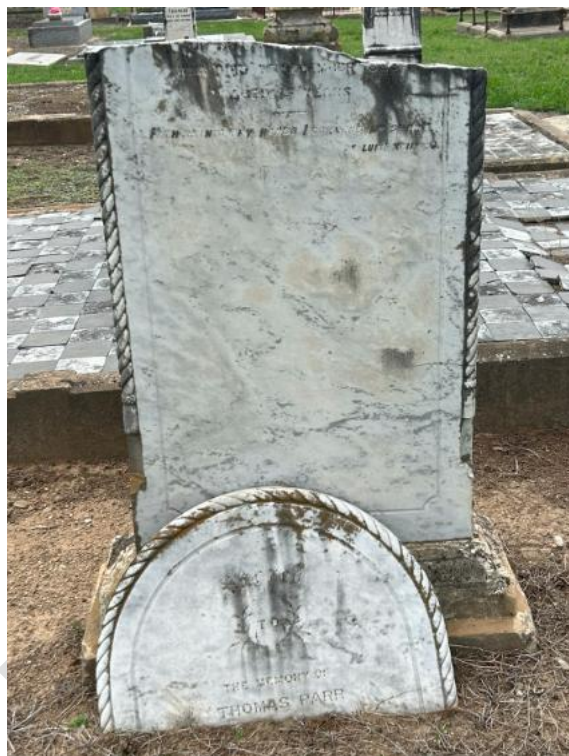
Figure 79: Example of a marble monument that has fractured resulting in the top portion breaking off
