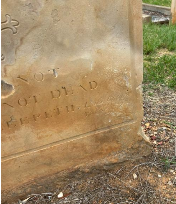
Figure 82: Example of rising damp in sandstone
