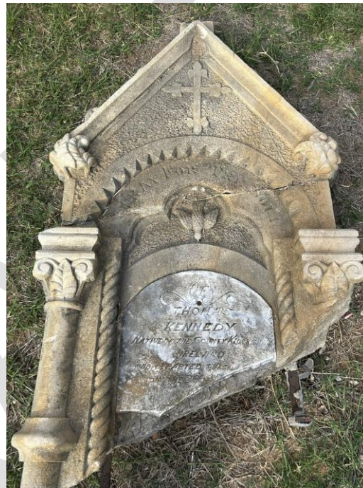
Figure 73: An example where the stone has fractured, leaving the monument in pieces
