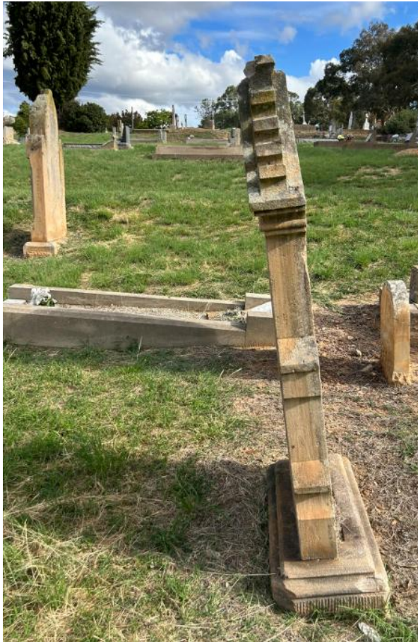
Figure 96: A sandstone monument leaning
