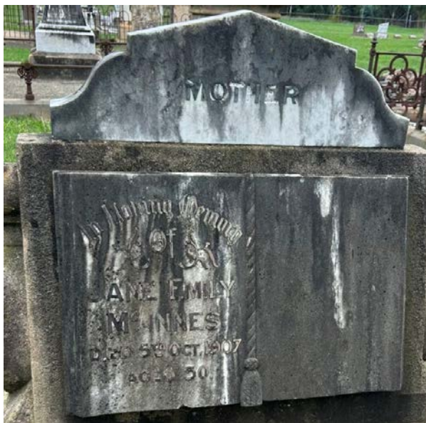
Figure 76: An example of the significant discolouration of a marble element
