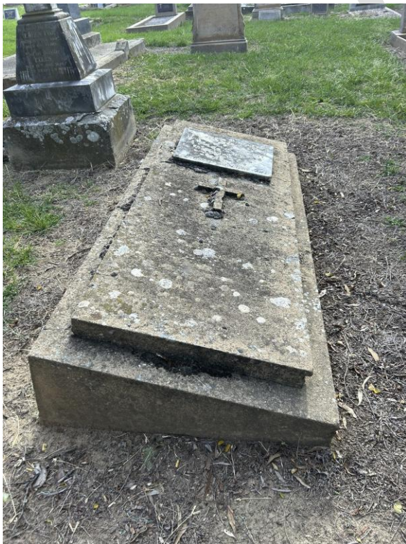
Figure 92: Example where subsidence is causing the grave to sink
