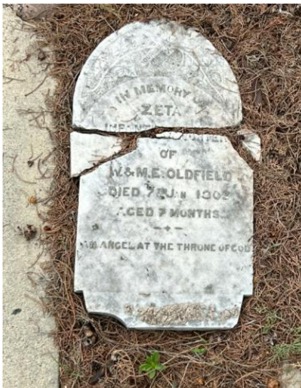
Figure 78: Example where a marble monument has fractured but been reassembled on the grave floor
