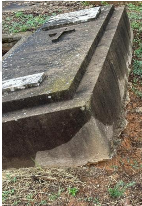
Figure 93: Example of subsidence leading to sinking of burial sites
