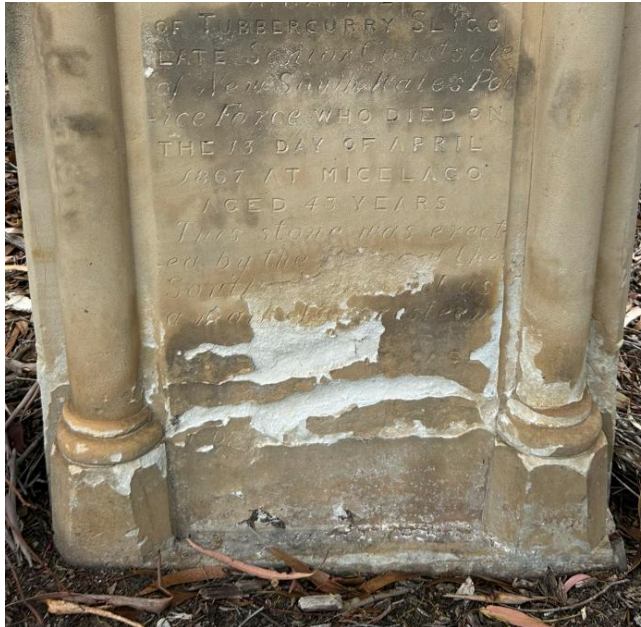
Figure 74: An example of spalling which has resulted in the loss of the stone surface
