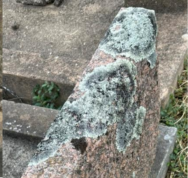
Figure 81: Biological growth on a granite headstone
