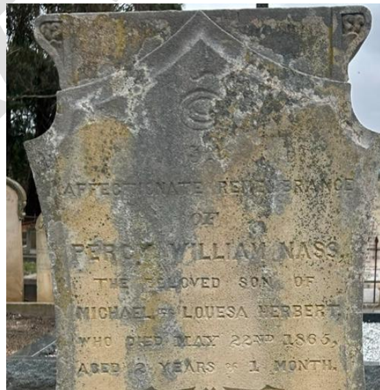
Figure 69: Sandstone discoloration resulting from biological growths
