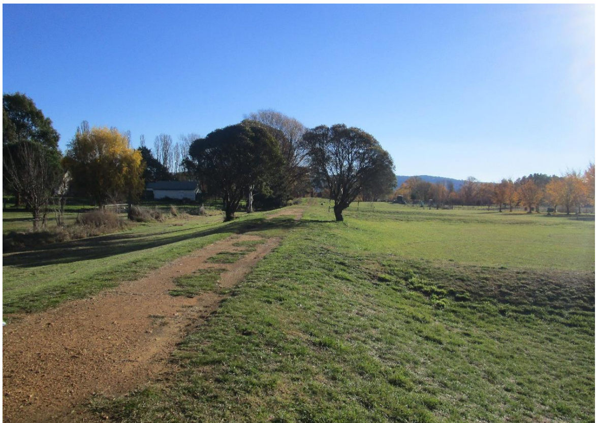
Figure 1-2 View of a section of the existing Turallo Terrace Levee, looking west
