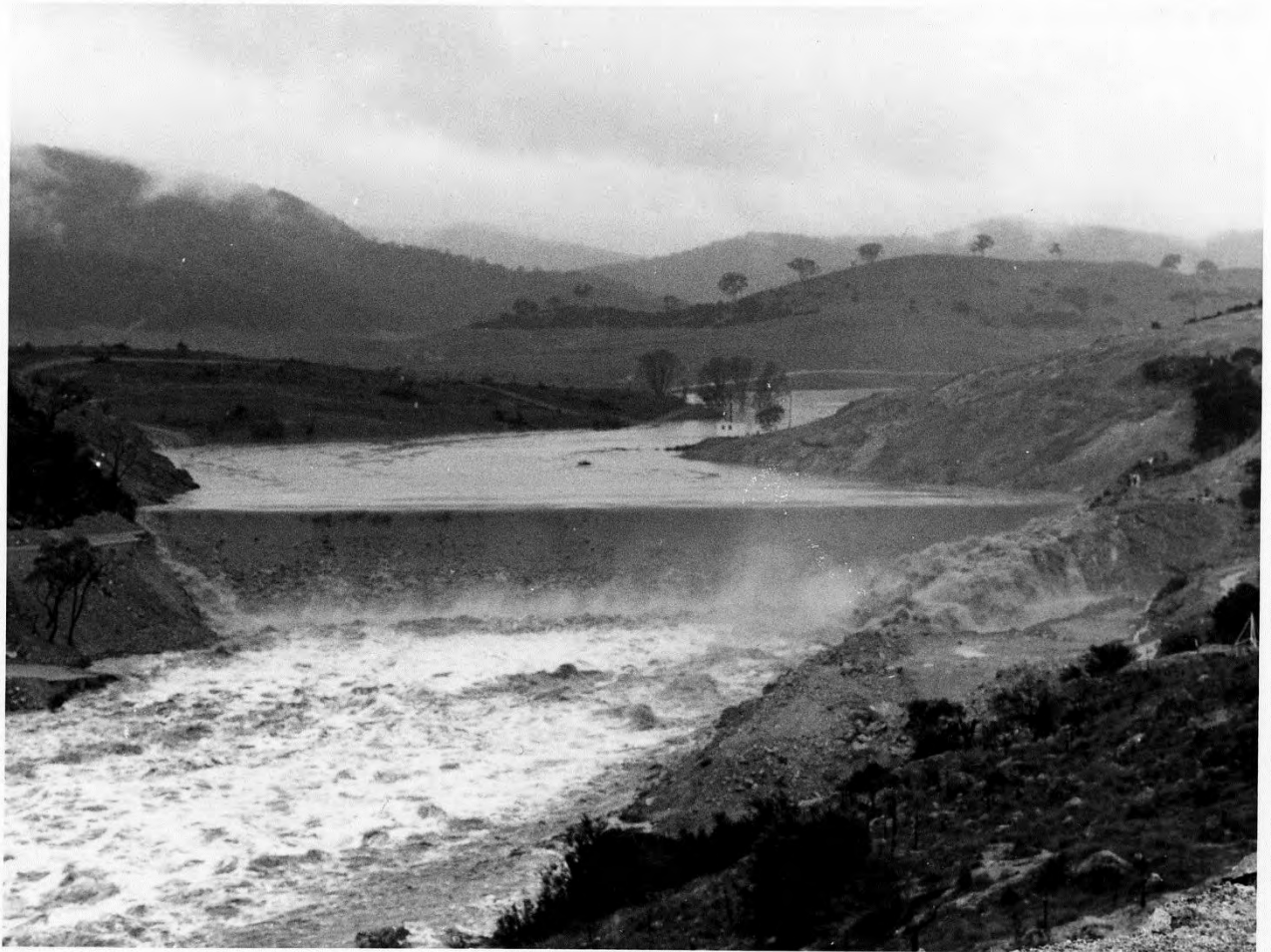
Plate B3.3 – Floodwater spilling over the partially constructed Googong Dam wall (Source: ArchivesACT )
