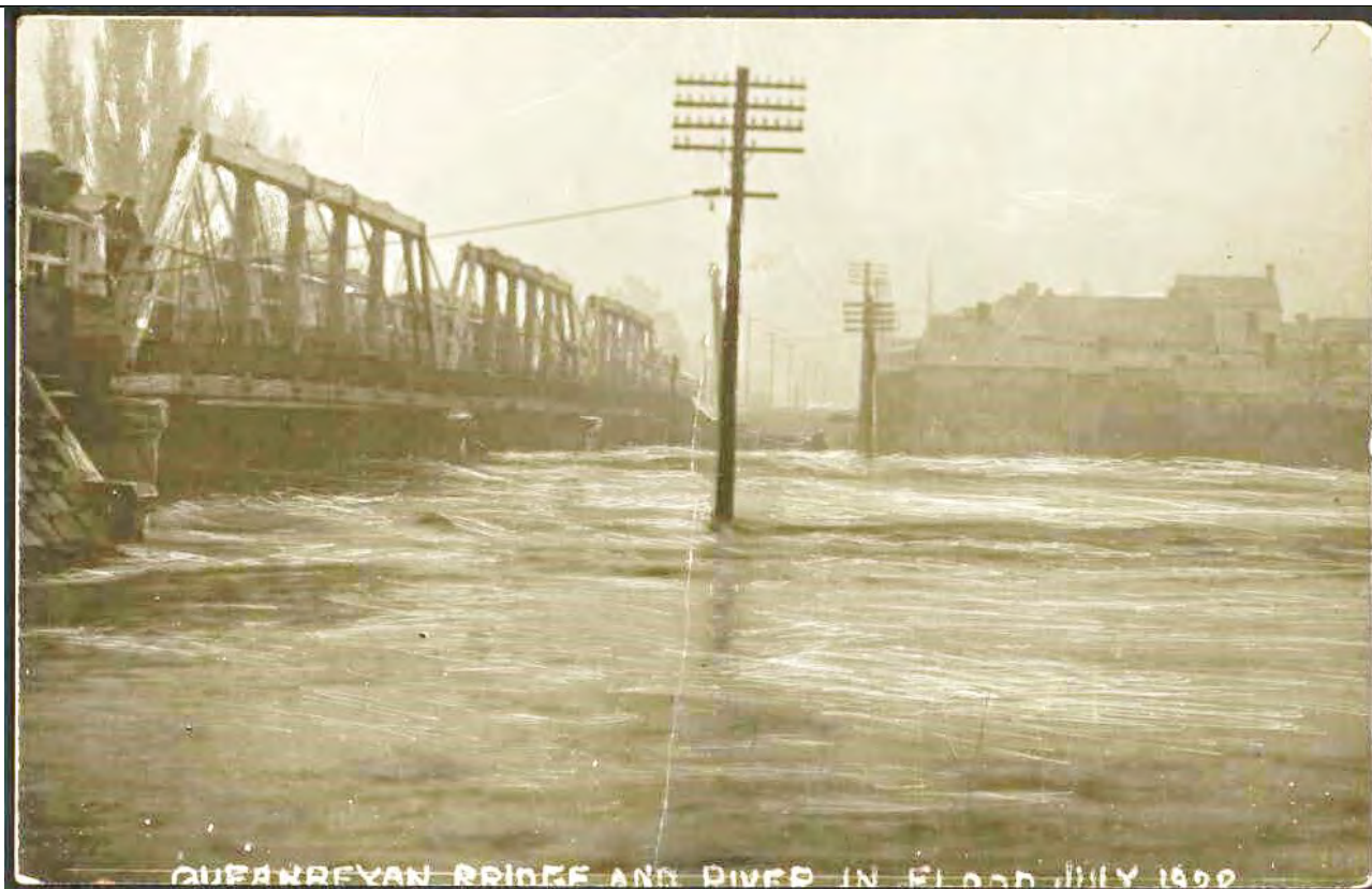
Plate B1.1 – Queanbeyan River downstream of old Kings Highway bridge.
