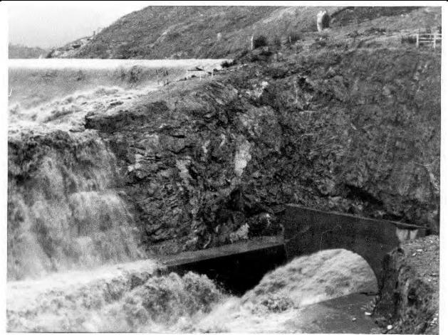
Plate B3.5 – Floodwater spilling over the partially constructed Googong Dam wall (Source: ArchivesACT)
