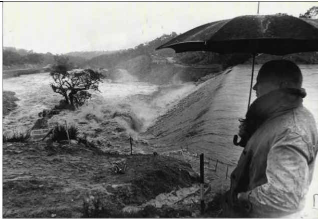
Plate B3.1 – Floodwater spilling over the partially constructed Googong Dam wall (Source: The Queanbeyan Age )
