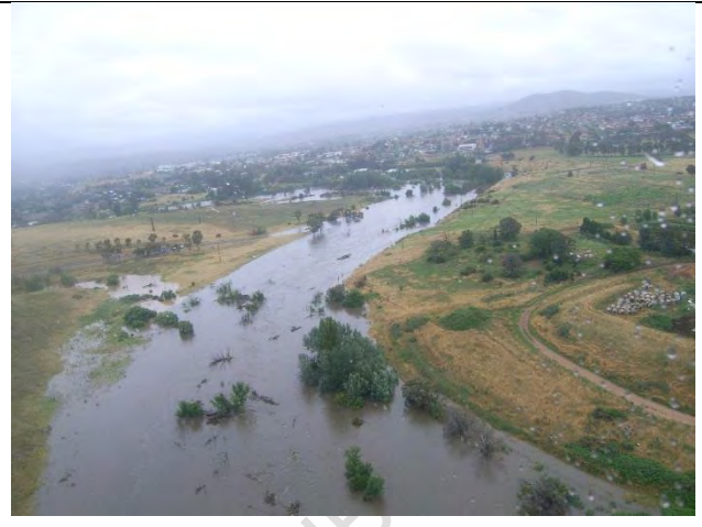
Plate B4.2 – 9/12/10 10:05 hours – Oaks Estate Road crossing of Molonglo River (road is submerged) (Source: NSW SES)
