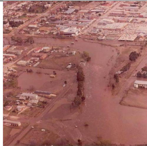
Plate B2.2 – Looking west across Queanbeyan River in vicinity of Morisset Street (Source: Council)
