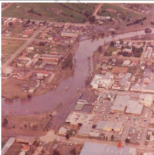
Plate B2.5 – Looking south along Queanbeyan River in vicinity of Queens Bridge (Source: Council)
