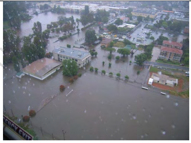
Plate B4.4 – 9/12/10 10:18 hours – Riverside Sporting Facility submerged by floodwater (Source: NSW SES)
