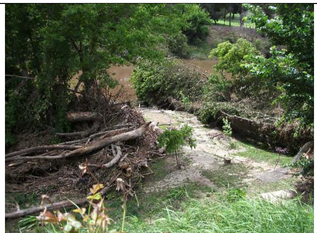
Plate B4.36 – 10/12/2010 – Build-up of debris on western bank of Queanbeyan River at eastern end of Hayes Street (Source: NSW SES)
