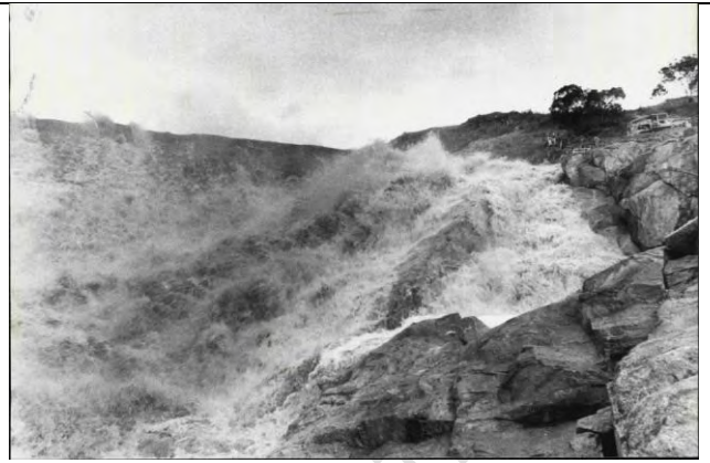
Plate B3. 2 – Floodwater spilling over the partially constructed Googong Dam wall (Source: The Queanbeyan Age )
