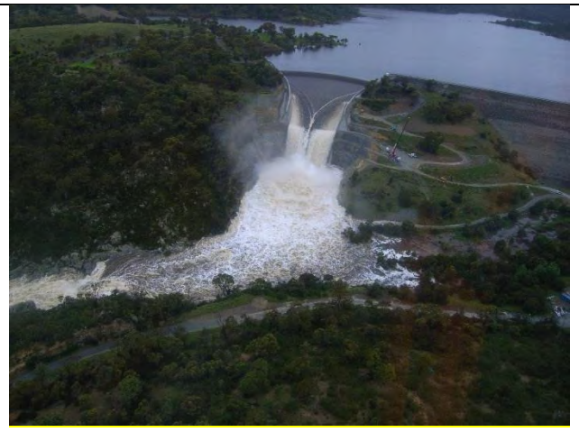
Plate B4.12 – 9/12/10 10:40 hours – Googong Dam Spillway (Source: NSW SES)
