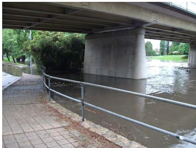
Plate B4.21 – 9/12/10 07:00 hours – Queens Bridge stream gauge (Gauge height 6.4 m) (Source: NSW SES)
