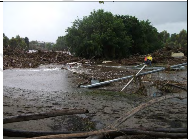
Plate B4.40 – Build-up of debris against Morisset Street bridge (Source: NSW SES)
