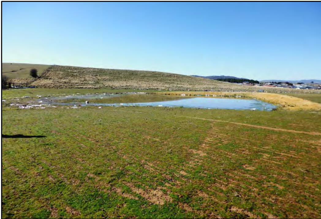
Photo 17: Dam in the north western portion - scattered rubbish from landfill
