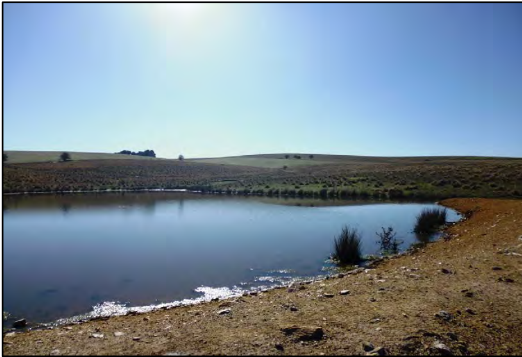
Photo 11: Dam in central portion
