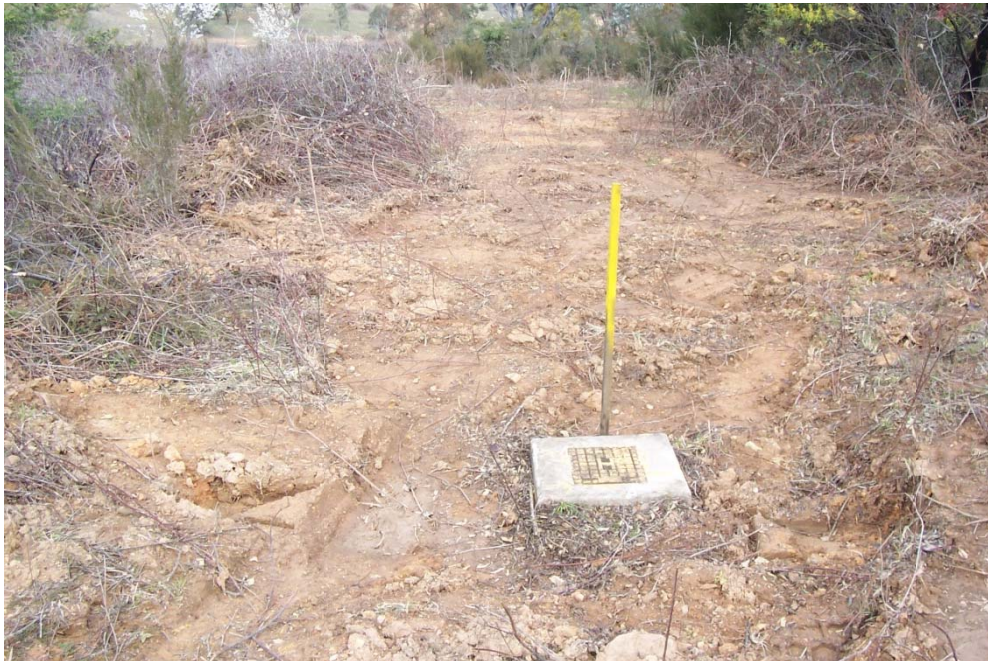
Photograph 2: Existing fire hydrant on the 375mm dia water rising main in the proposed Ellerton Drive reserve
