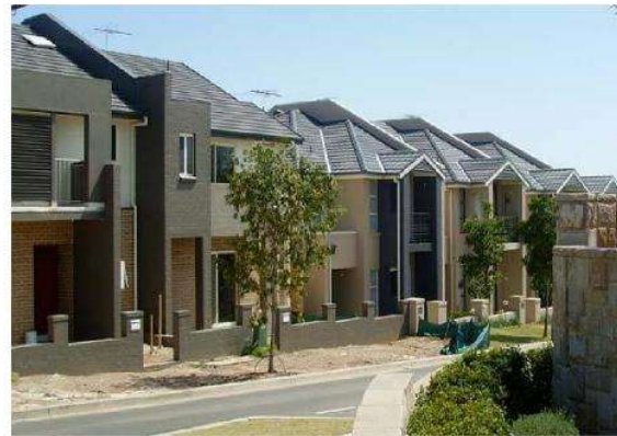
Broken wall planes and articulation
