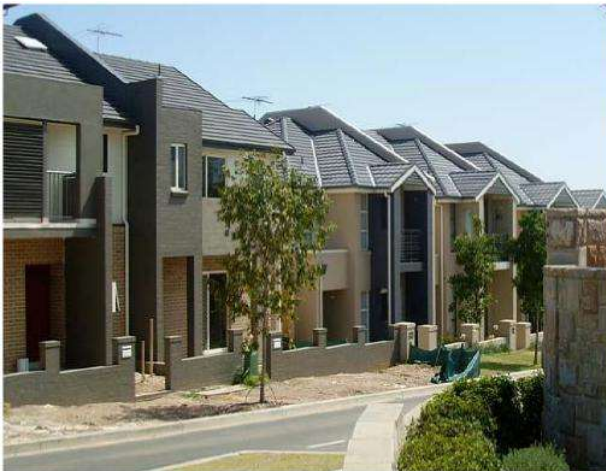
Broken wall planes and articulation
