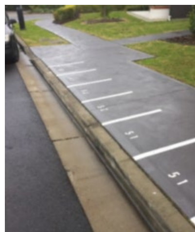
Figure 3 Good practice example of defined waste service collection points (NSW EPA, 2019)
