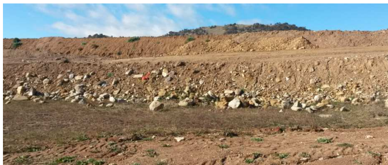
Photos 1 to 4 (above) – 18/7/14 – View of road fill and fill stockpiles on north-western side of the site.
