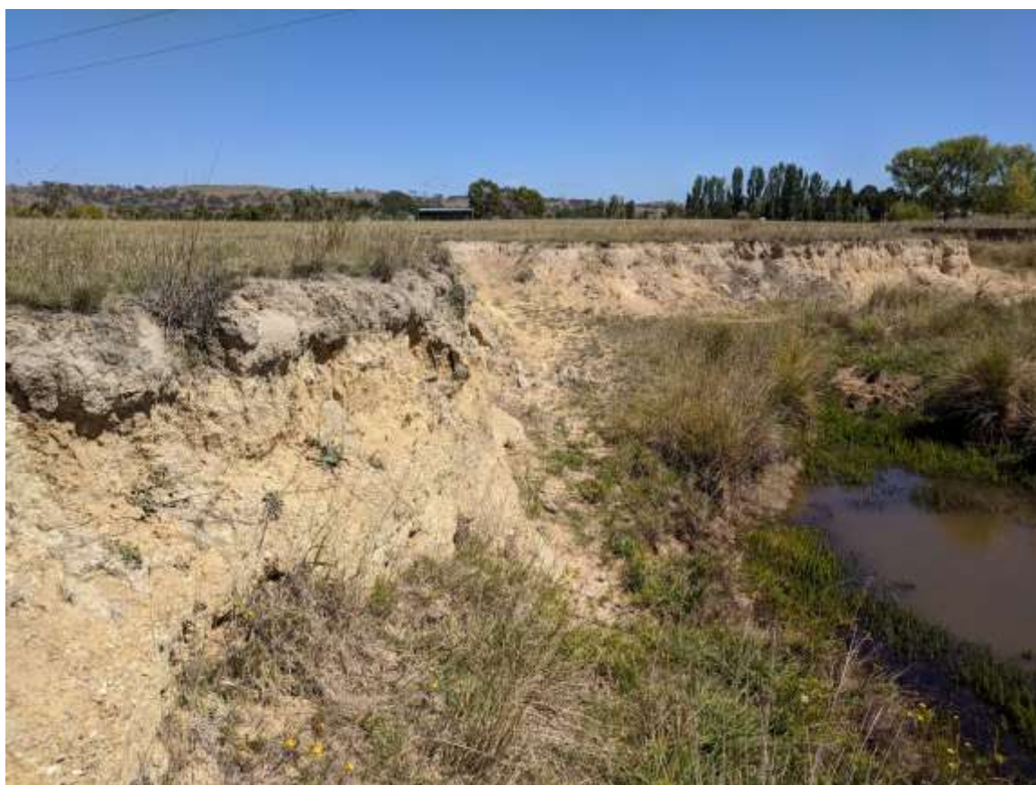
Figure 6-2: Example 2 of erosion within Church Creek
