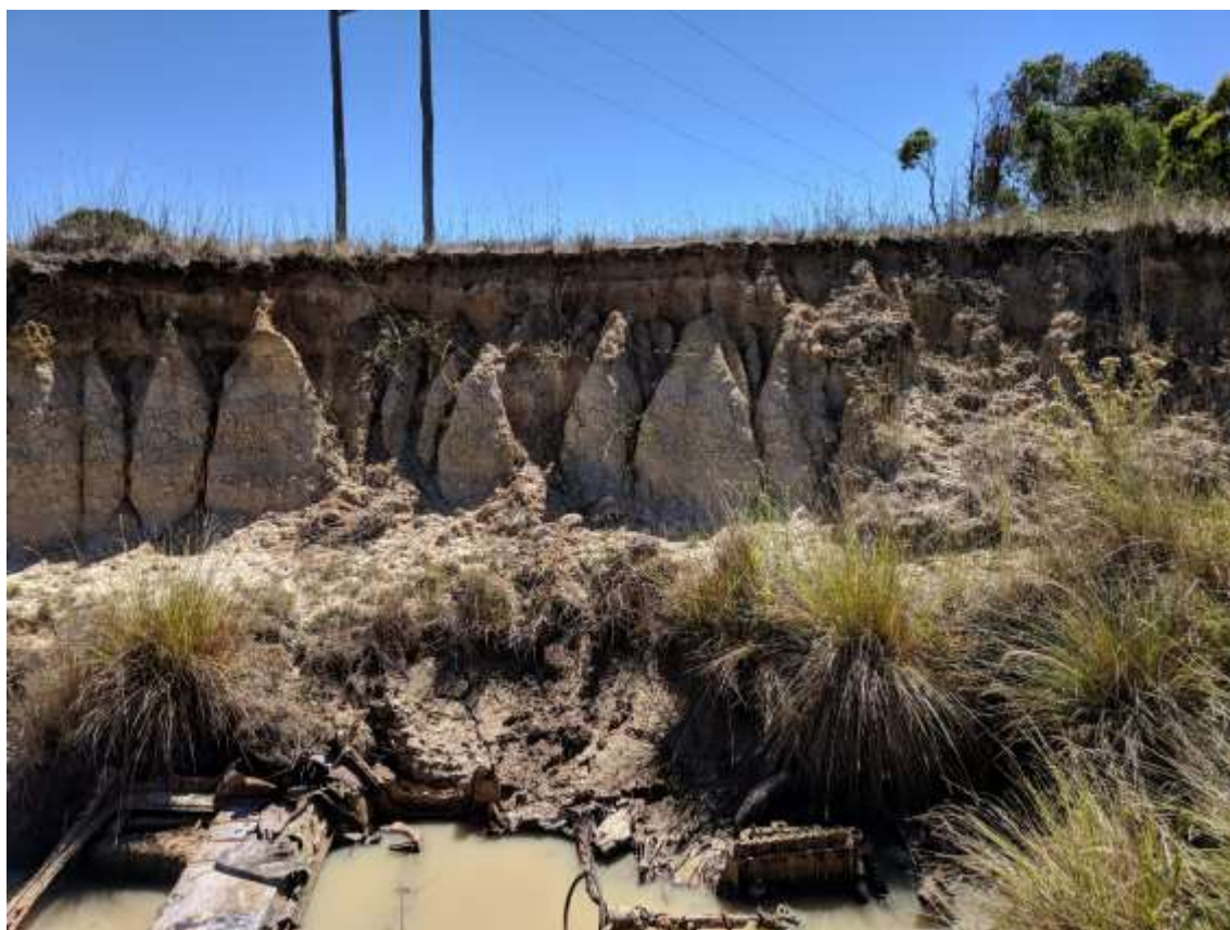
Figure 6-1: Example 1 of erosion within Church Creek
