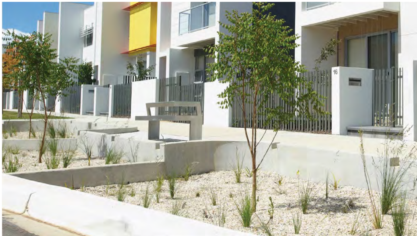
Figure 6-2: Example of constructed raingarden
