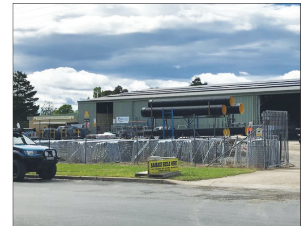
Figure 13 – Industrial development on southern side of Gillamatong Lane
