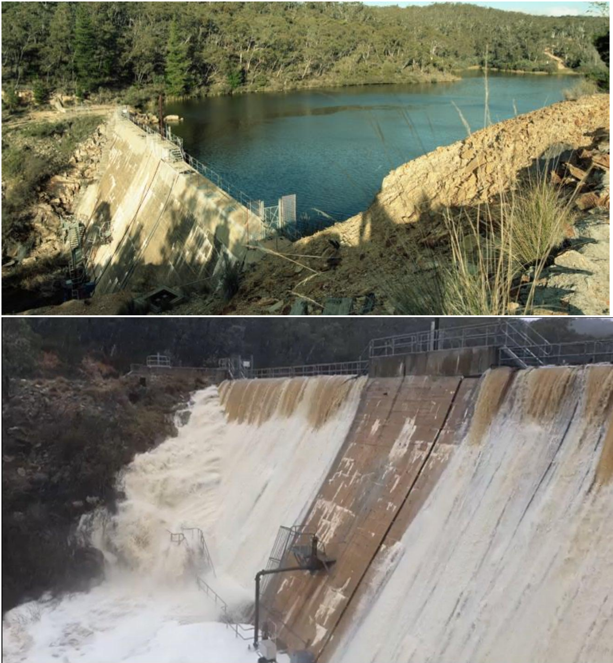
Figure 2-2: Images of Captains Flat dam in dry (2014) and overtopping (2020) conditions,
