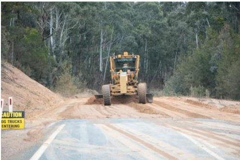
Road Grader at Nerriga Road. I
