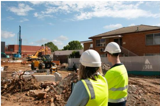
WHS officers inspecting a worksite.
