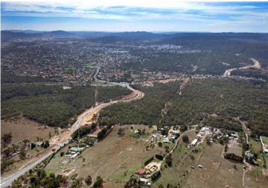
Cooma Road Realignment.
